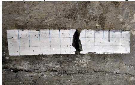
Figure 2. Failure pattern of the 0% sample specimen
